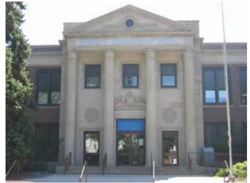
Everett Elementary School at 11th & C Sts.
